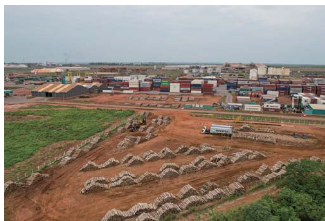
Rail Depot in Rondonópolis, Mato Grosso, Brazil. Photo: teakrc
